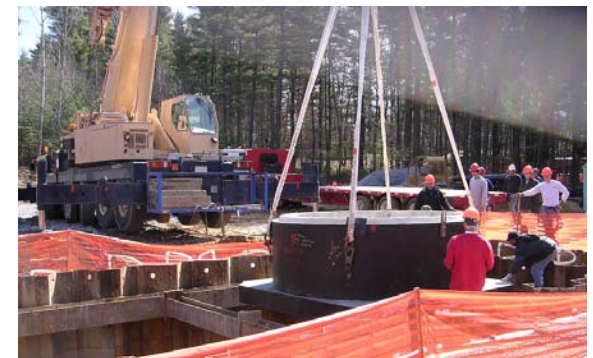
Bottom: Tokanel Drive Pump Station Construction
