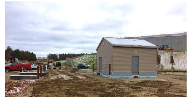
Top: Webb Drive Pump Station Construction
