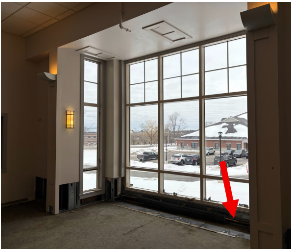
FIGURE 1 DRYWALL REMOVED AT BUMP-OUTS
