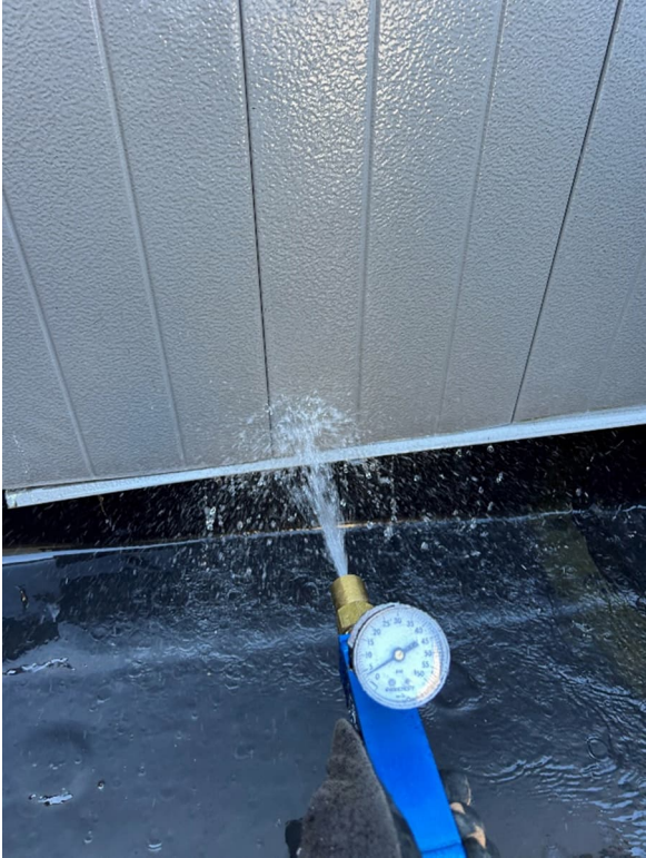
FIGURE 3 TESTING THE ROOF TO WALL DETAIL ON THE DORMER
