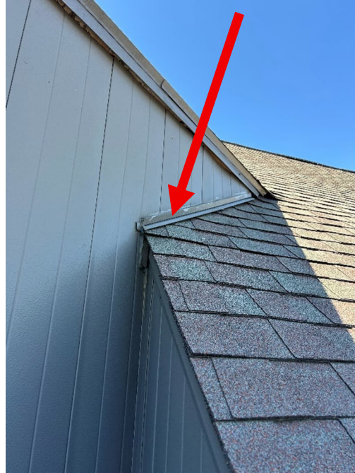
FIGURE 10 RIGHT SIDE OF DORMER (HIGH): NO LEAK
