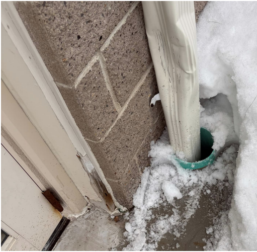
FIGURE 22 DAMAGED DOWNSPOUT
