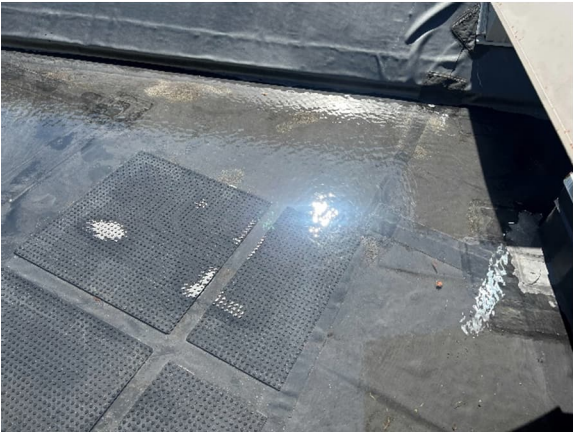
FIGURE 20 INFORMAL ROOF PONDING TEST
