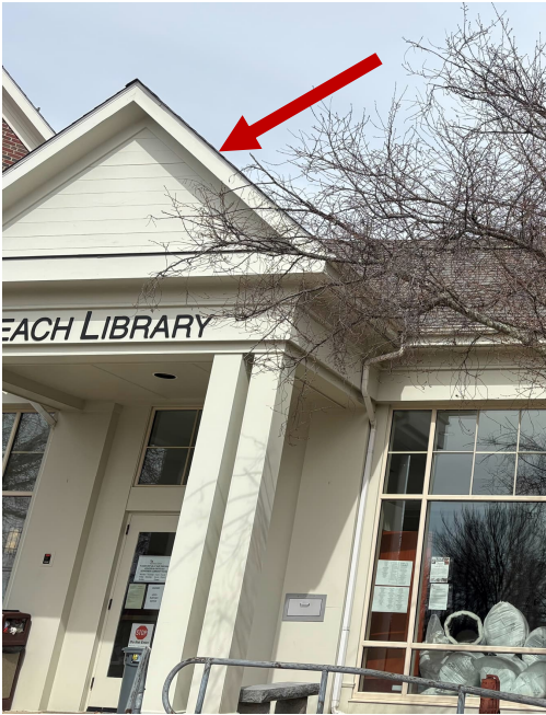
FIGURE 1 VENTED DORMER OVER ENTRY
