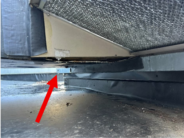
FIGURE 8 TESTING IN PROGRESS
