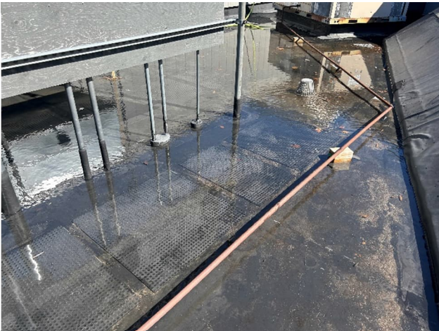
FIGURE 21 INFORMAL ROOF PONDING TEST
