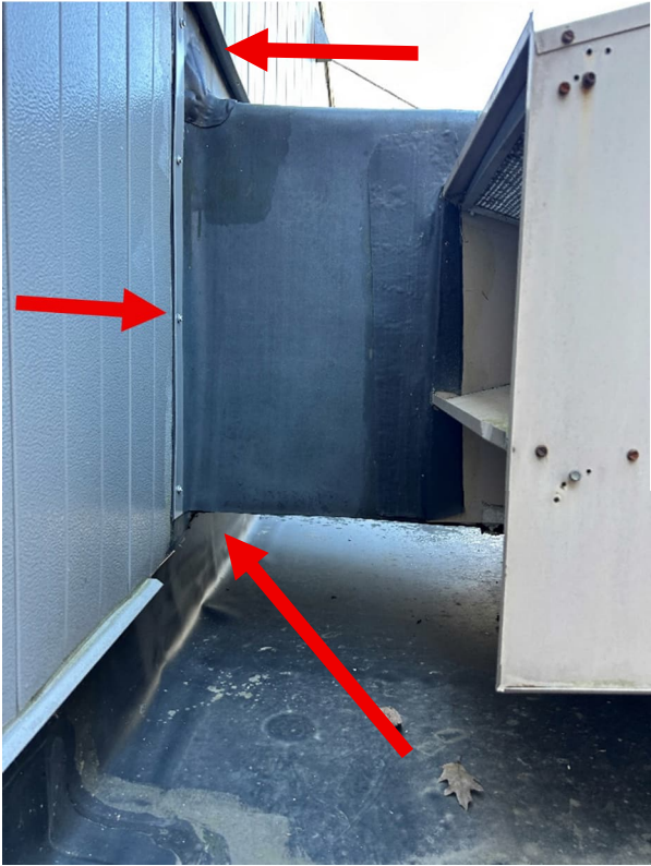
FIGURE 7 DUCT TO WALL DETAIL: NO LEAK
