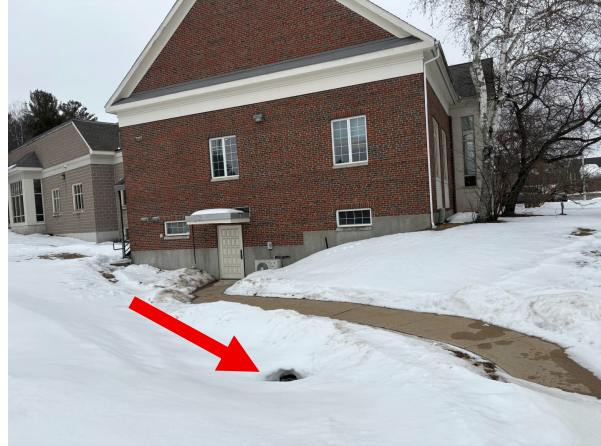
FIGURE 10 SWALE WITH DRAIN
