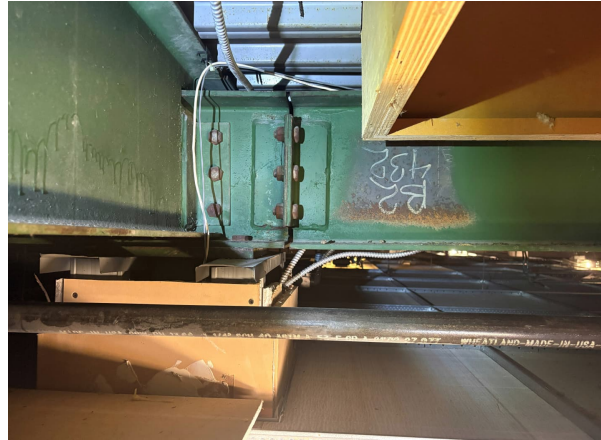
FIGURE 13 STRUCTURAL STEEL FROM THE ORIGINAL FLAT ROOF.
