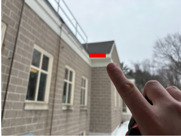
FIGURE 9 MISSING GUTTER
