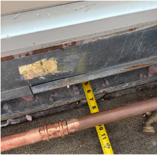
FIGURE 3 INSULATION SPACE BEHIND HORIZONTAL HEAT PIPE
