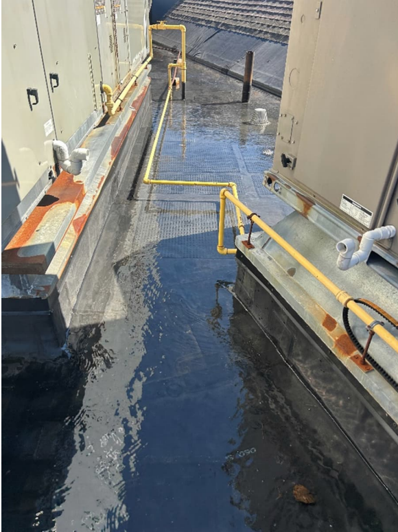
FIGURE 18 INFORMAL ROOF PONDING TEST
