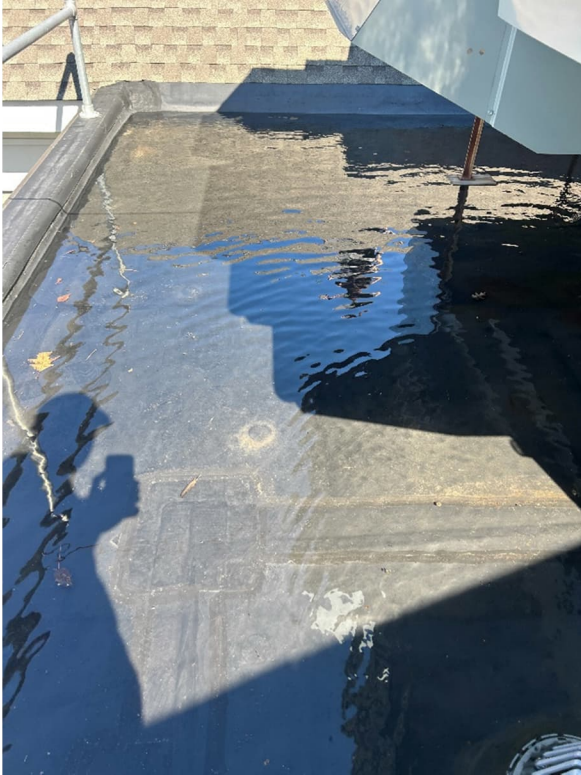
FIGURE 19 INFORMAL ROOF PONDING TEST
