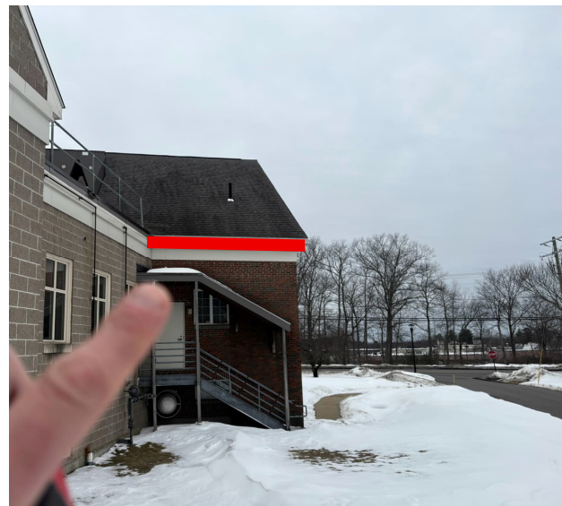
FIGURE 8 MISSING GUTTER
