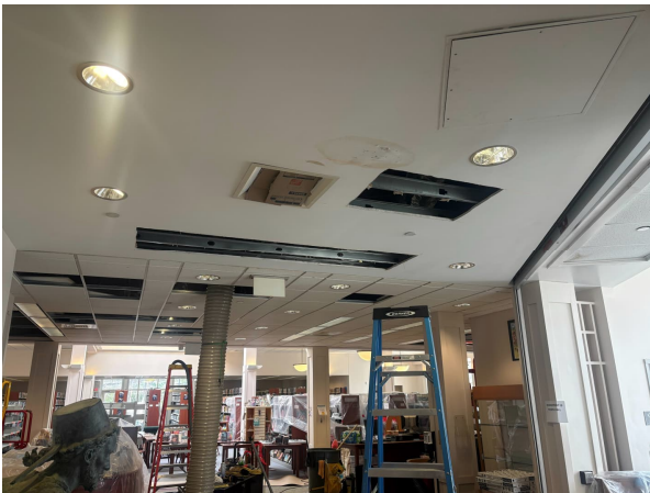
FIGURE 3 HOLES CUT IN GYP CEILING
